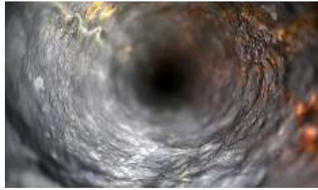
Real life problem 2 Corrosion of Piping
